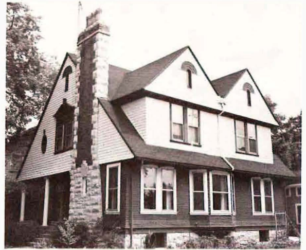
8. THE HOLDEN HOUSE 905 Church Street
