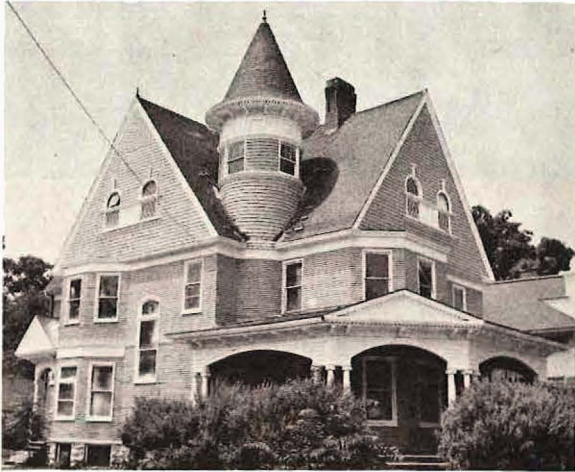
5. THE PALEY HOUSE 802 Park Avenue
